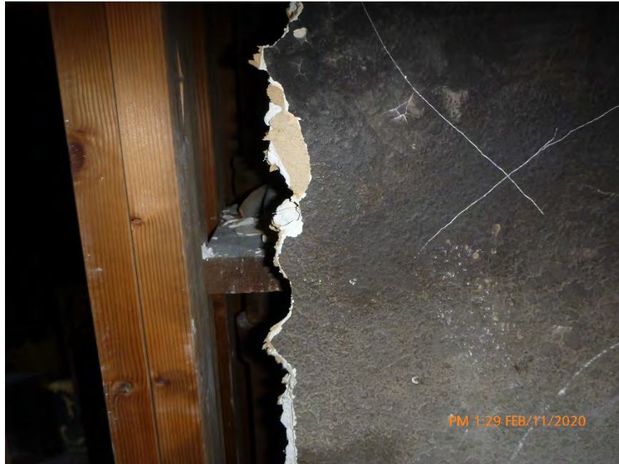
Photograph 9: February 11, 2020, at approximately 1:29 PM – View of textured drywall on a hallway wall in Unit 1. The material was sampled and later determined to contain 2% Chrysotile Asbestos by the point count method using polarized light microscopy.
