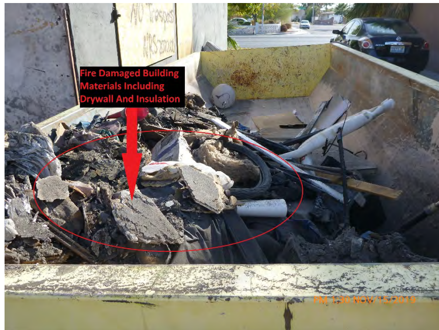
Photograph 2: November 15, 2019, at approximately 1:30 PM - View of fire damaged building materials in a 16 cubic yard dumpster. The debris was in a dry condition with no evidence of moisture.
