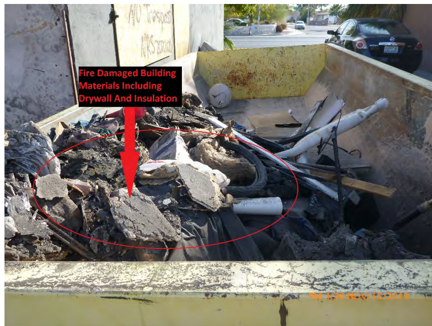
Photograph 2: November 15, 2019, at approximately 1:30 PM - View of fire damaged building materials in a 16 cubic yard dumpster. The debris was in a dry condition with no evidence of moisture.
