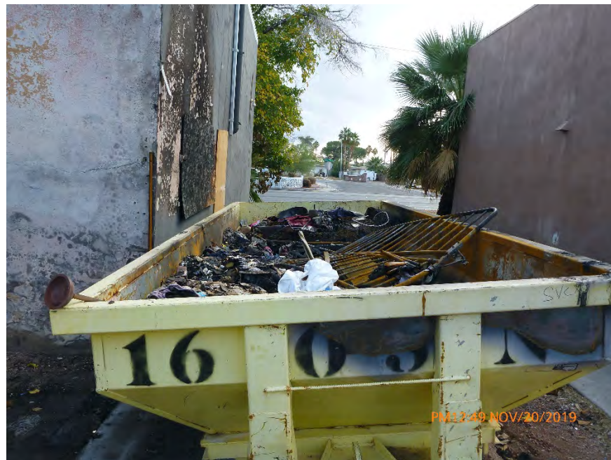
Photograph 23: November 20, 2019, at approximately 12:49 PM - View of the 16 cubic yard dumpster which contains ACWM. The dumpster remains uncovered and is not posted with asbestos warning signs.
