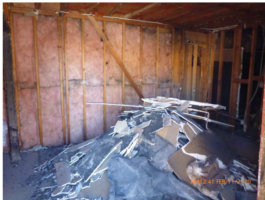
Photograph 2: February 11, 2020, at approximately 12:41 PM - View of Asbestos-Containing Waste Material (ACWM) inside of the north room of Unit 1. The ACWM was in a dry condition with no evidence of moisture. Textured drywall, including acoustic ceiling texture, had been removed from all of the walls and ceilings. The texture on the walls and ceilings were Regulated Asbestos-Containing Materials.
