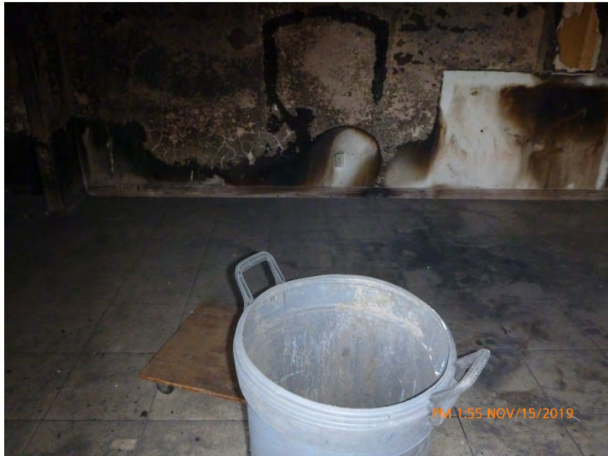
Photograph 6: November 15, 2019, at approximately 1:55 PM - View of a waste bin in the north room (Master Bedroom) of Unit 1. Note the lack of a significant amount of debris on the floor.
