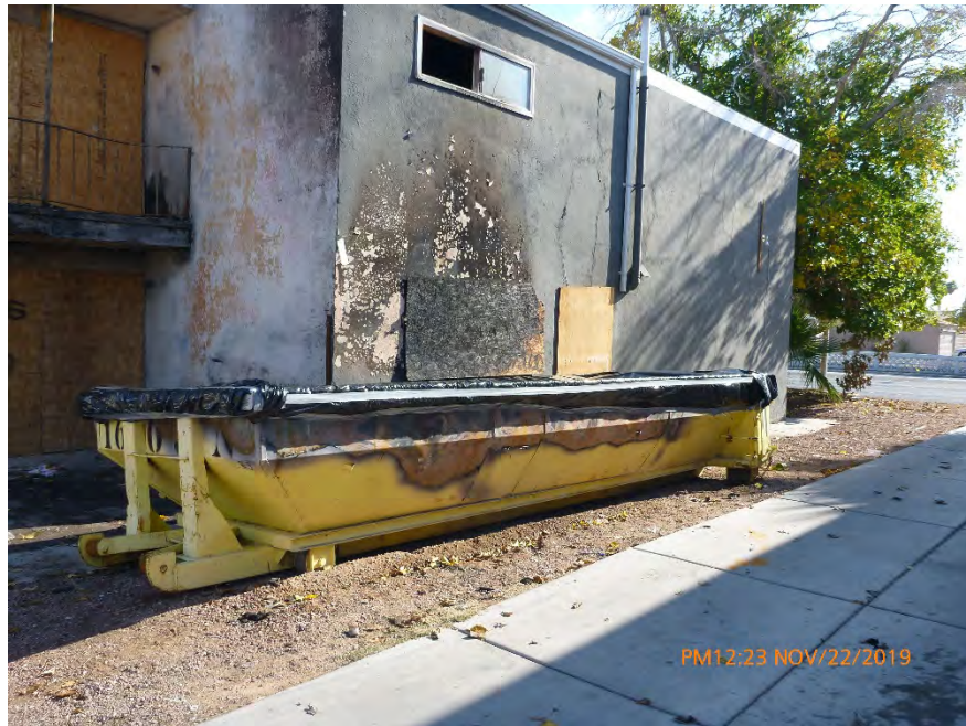
Photograph 26: November 22, 2019, at approximately 12:23 PM - View of the 16 cubic yard dumpster which contains ACWM. The dumpster is sealed but asbestos warning signs are not posted.
